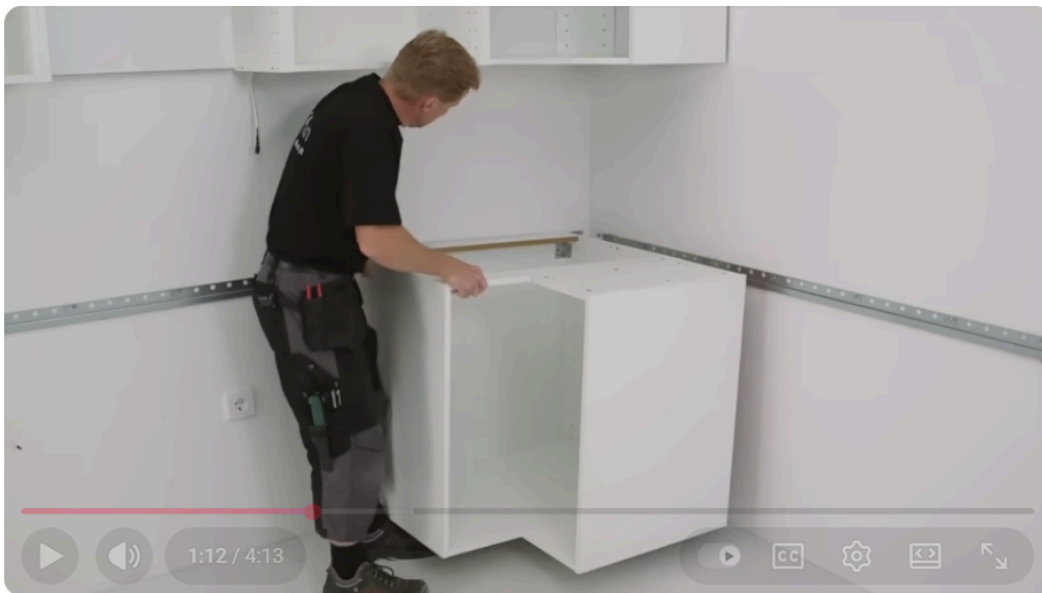
Figure 3b: Installing IKEA kitchen cabinets on a wall-mounted steel cleat. Screen-shot from IKEA METOD Kitchen Installation 3/7 - Installing the cabinets.
